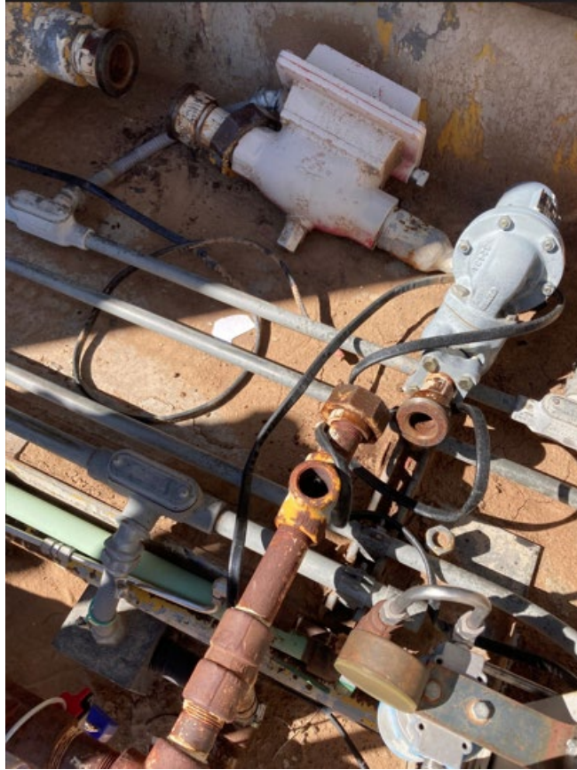
Caterpillar Engine Fuel Gas Line – Air Gapped
