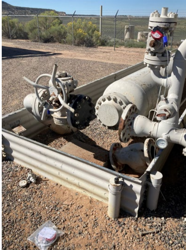
Caterpillar Engine Discharge - Air Gapped and Blind Flanged
